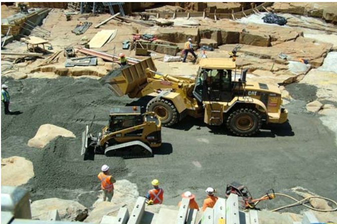
Above: Meander Dam foundation area showing placement and compaction of RCC.
